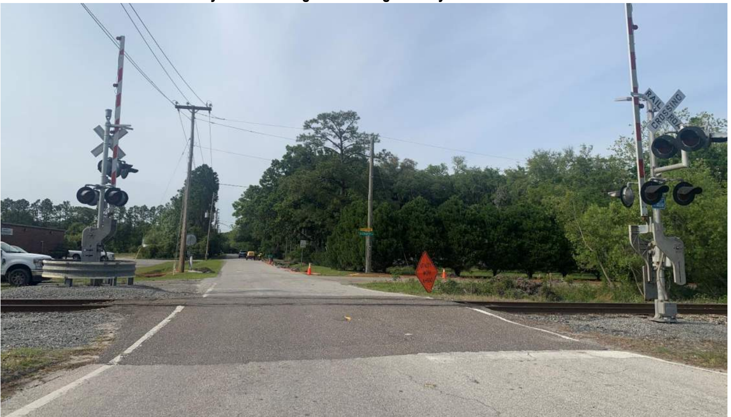
Southbound Friendly Road Looking North Along Friendly Road Towards Railroad Tracks
