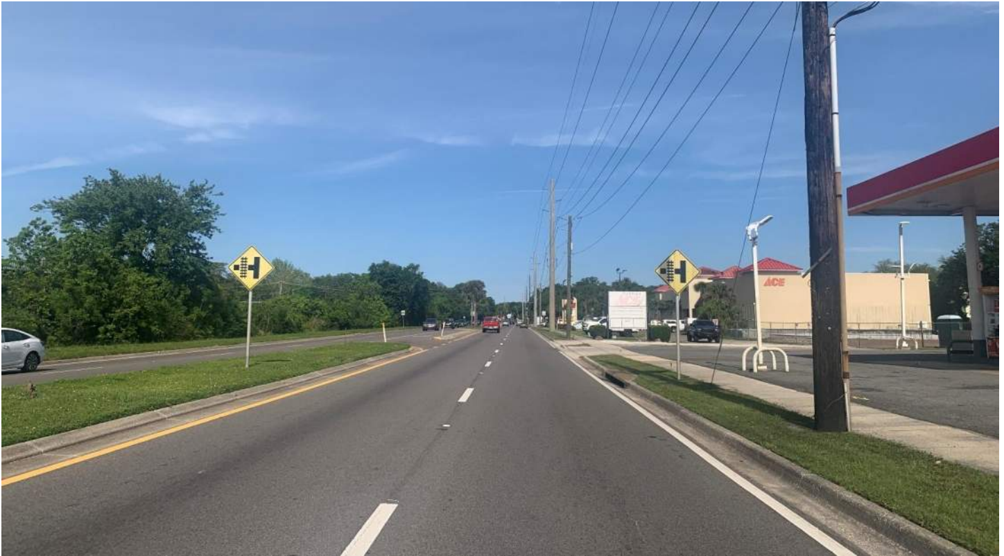
Intersection Warning Signs on Eastbound SR A1A Approaching Friendly Road
