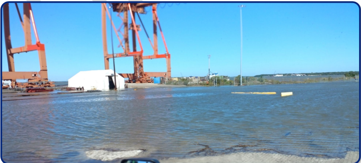
Figure 12 - Severe Flooding due to King Tides at Port of Fernandina
