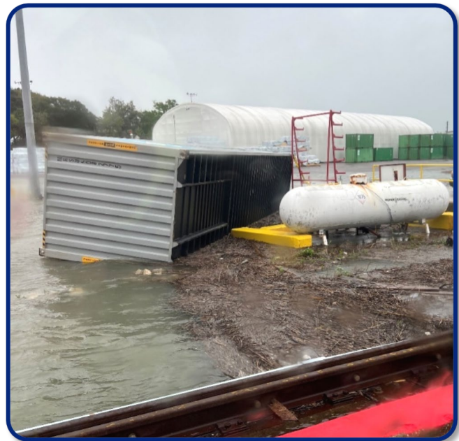
Source: Photo courtesy OHPA Staff, November 2022
